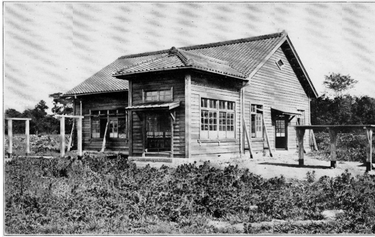
GYMNASIUM—Length 48 ft., width 36 ft.
